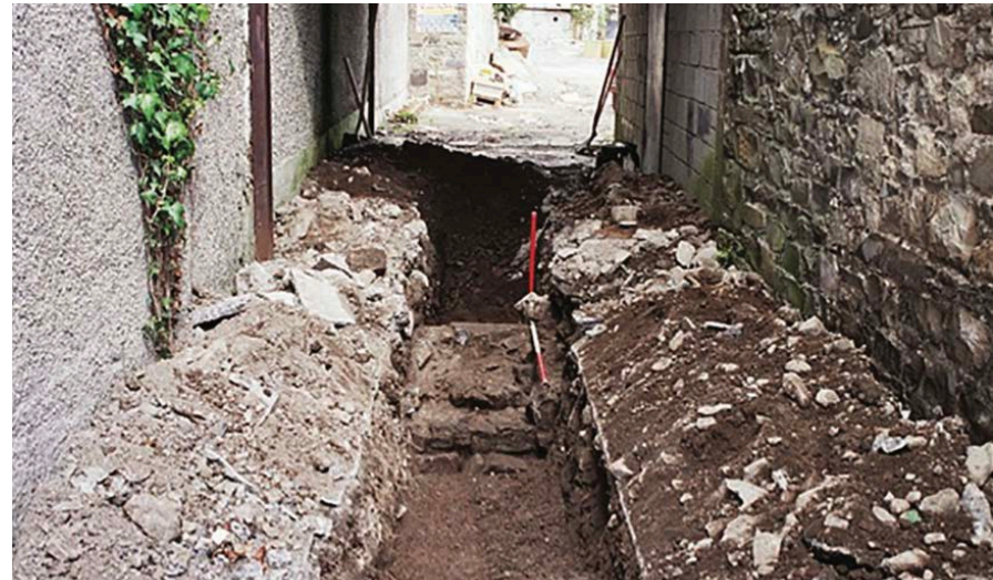
40. View towards medieval town wall base along south alignment.
