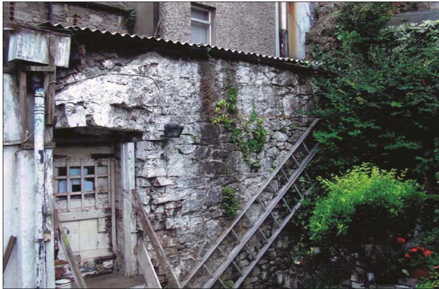
37. Upstanding wall at rear of 13 Ludlow Street (courtesy V Mulvany).
