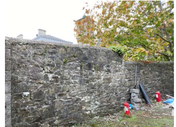
32. Southern alignment (internal) in yard.
