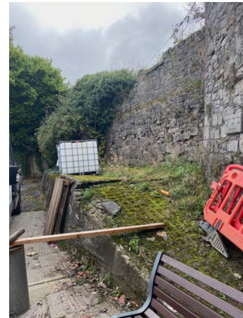
21. View along wall section towards bastion.
