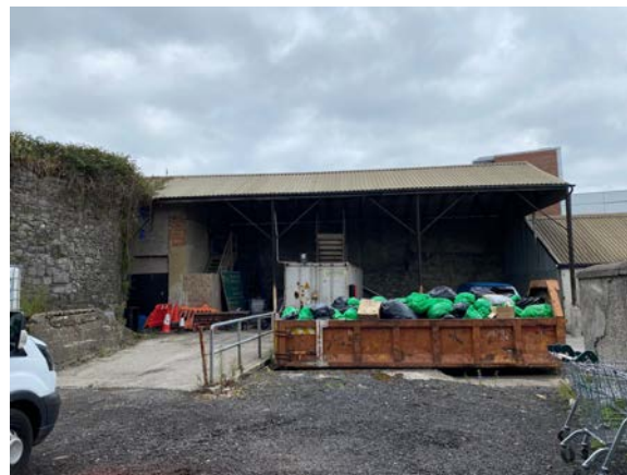
26. View towards MCC depot shed.
