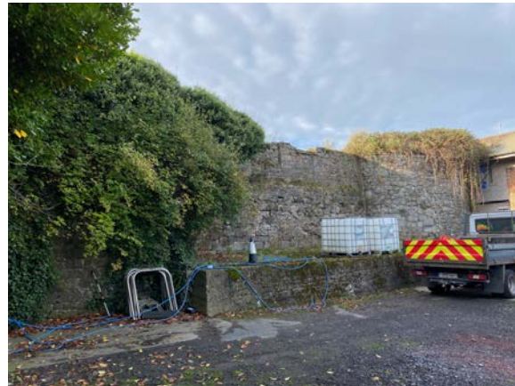
23. View along wall section towards bastion.
