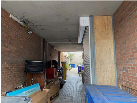
30. View along gated passage over wall circuit.
