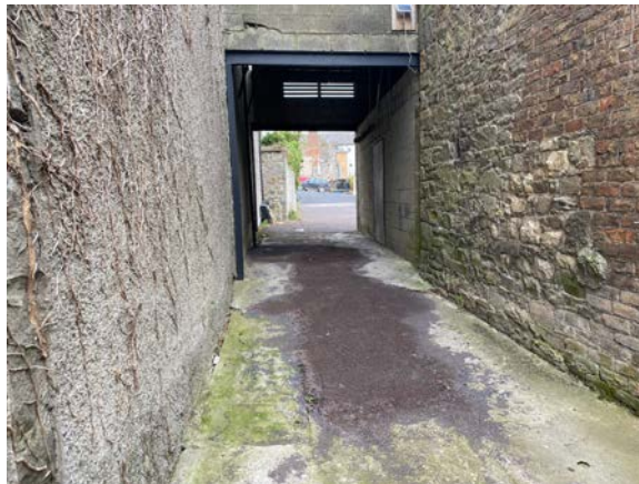
19. View along lane across wall alignment.
