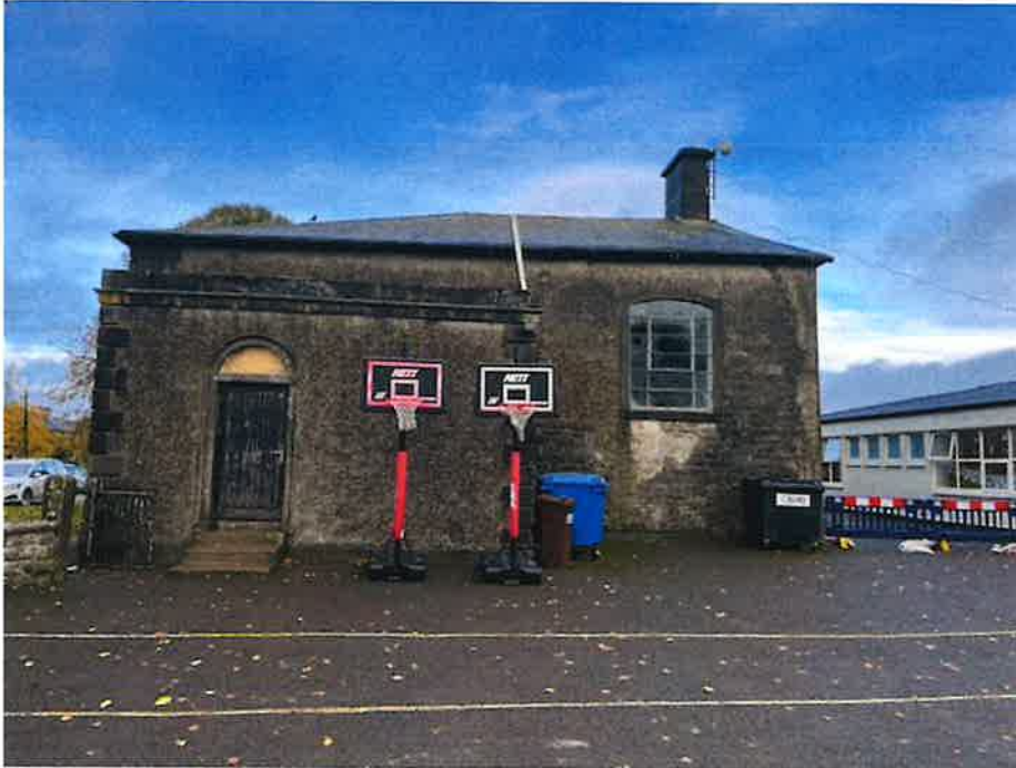
View of east wing elevation 1826 building with 1977 building to right.
