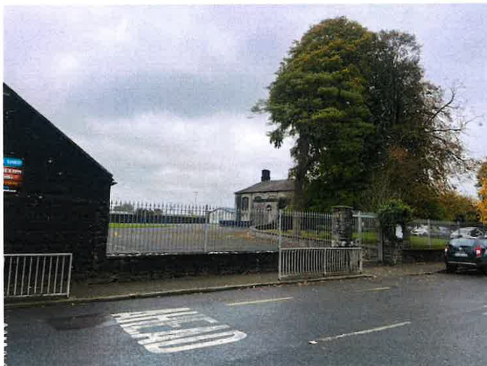
View of site from west on Church Road (1977 building visible behind).
