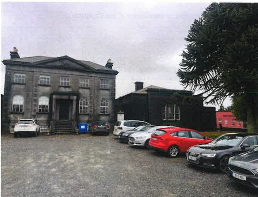
View of existing car park to front of 1826 building – proposed location of EV charger located approximately behind red car.
