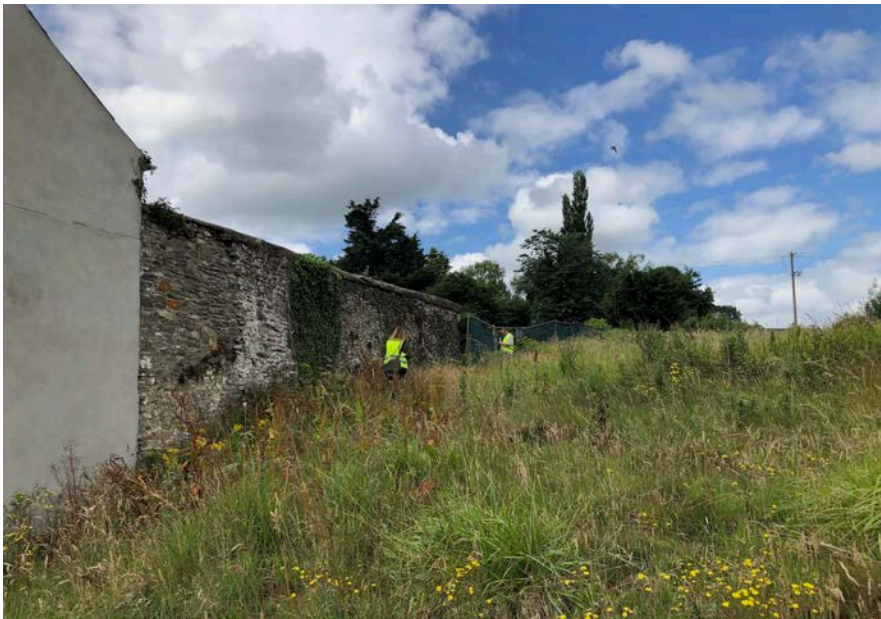
31. Carrying out survey along the wall circuit.
