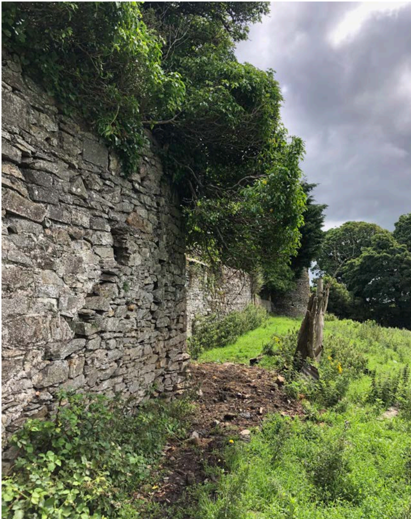
13. View along wall alignment to rear of Cannon Street.
