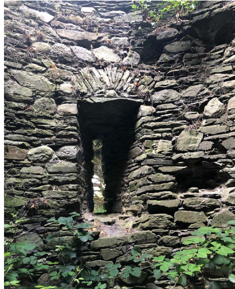
16: Detail of arrow loop embrasure to the mural tower.
