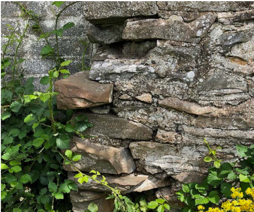
12. Detail of stone wall and concrete block infill.
