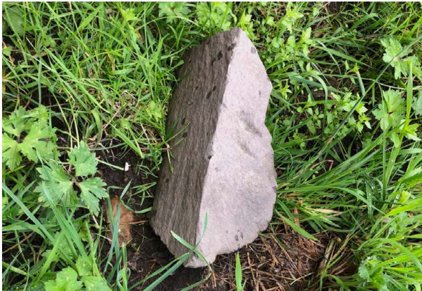
4. Detail of displaced building stone in field close to town wall.
