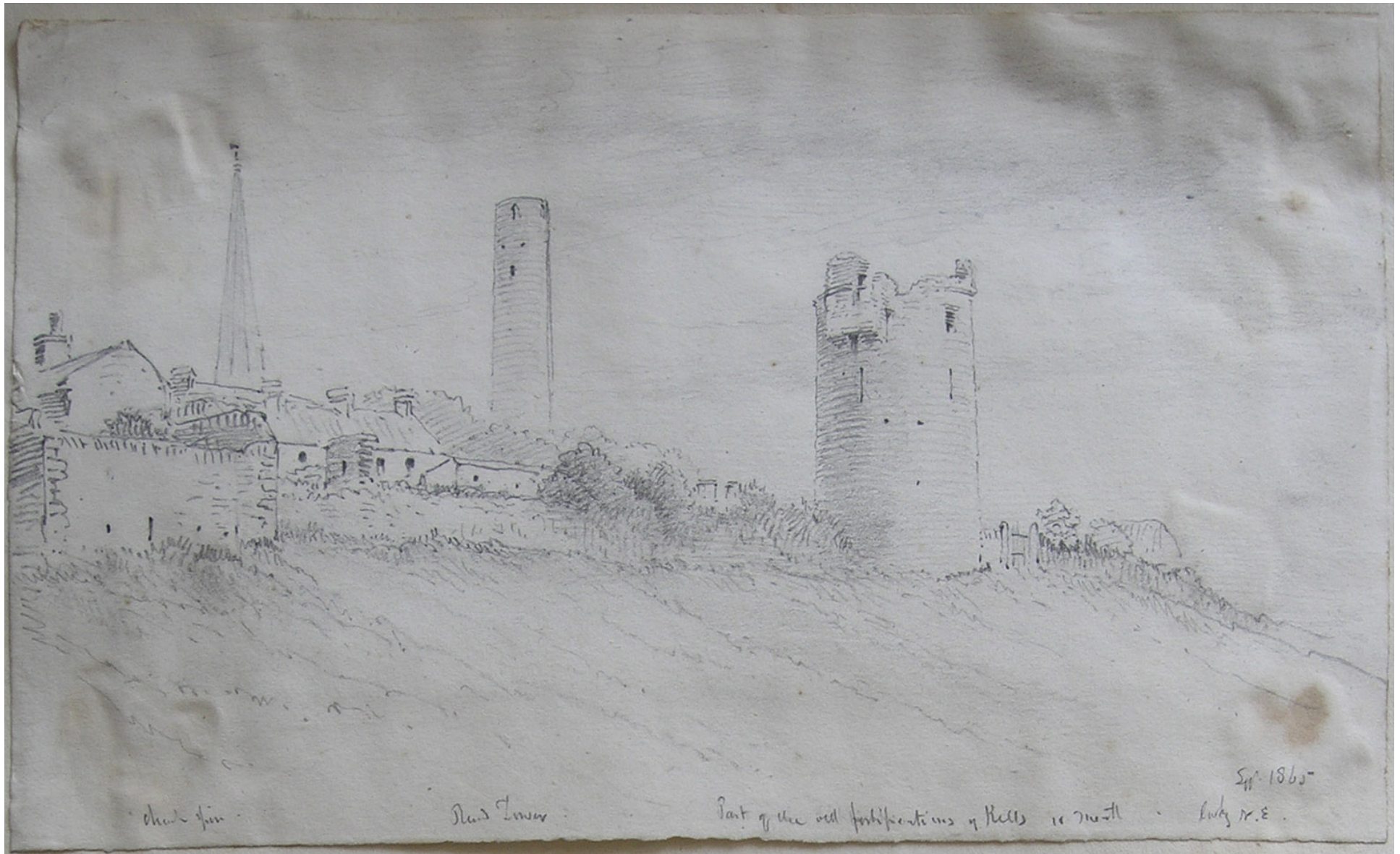
10.. GV Du Noyer view of 1865 showing the mural tower and town wall with the spire and round tower from the monastic site in the background. Note breakfront wall to LHS and vegetation, infill wall to 14 & 15 Cannon Street, machicolation and parapet to tower.
