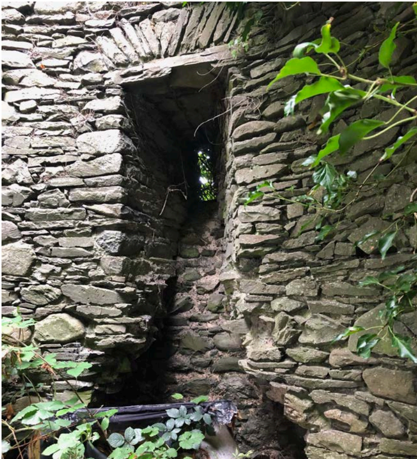
18. Detail of arrow loop embrasure to mural tower.
