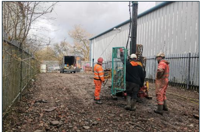
Rotary boring rig
