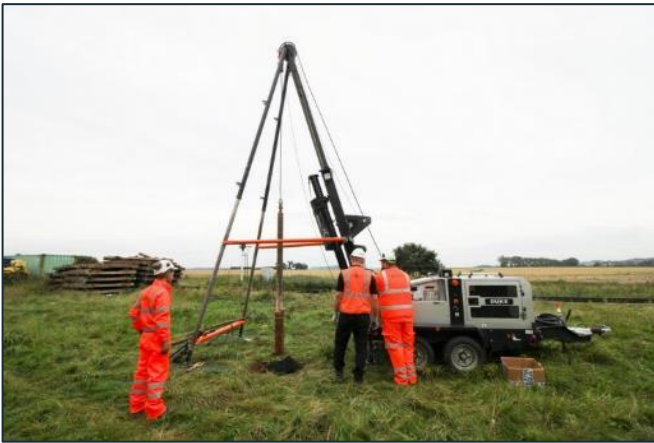
Cable percussion boring rig
