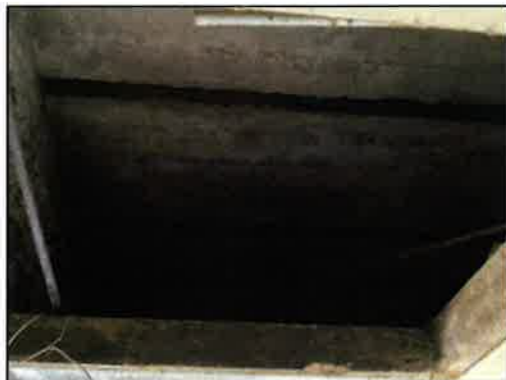
Photo - 52 In-situ concrete slab over Kitchen extension over disused railway lines
