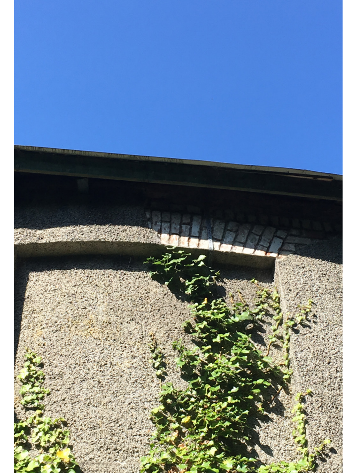
The cement Pebble dash render covering brickwork.
