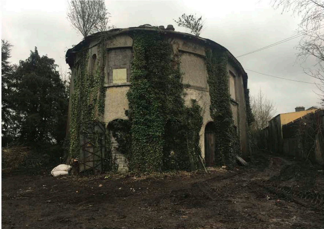
Current Condition of St. Patrick's Classical School.
