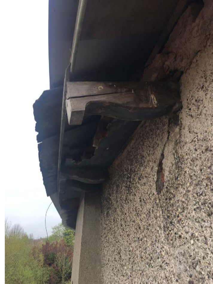
Rafters supporting the Slate roof.
