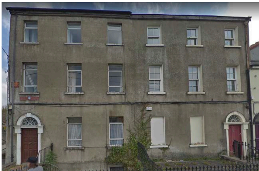
End-of-terrace three-bay three-storey house over basement on Academy Street
