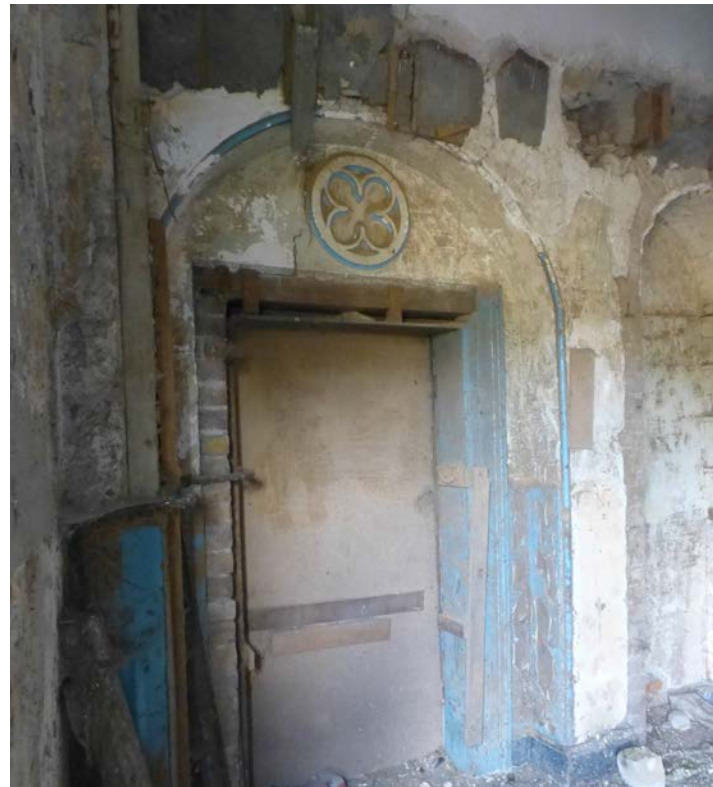
Large decorated motifs similar in style to the roof trusses.
