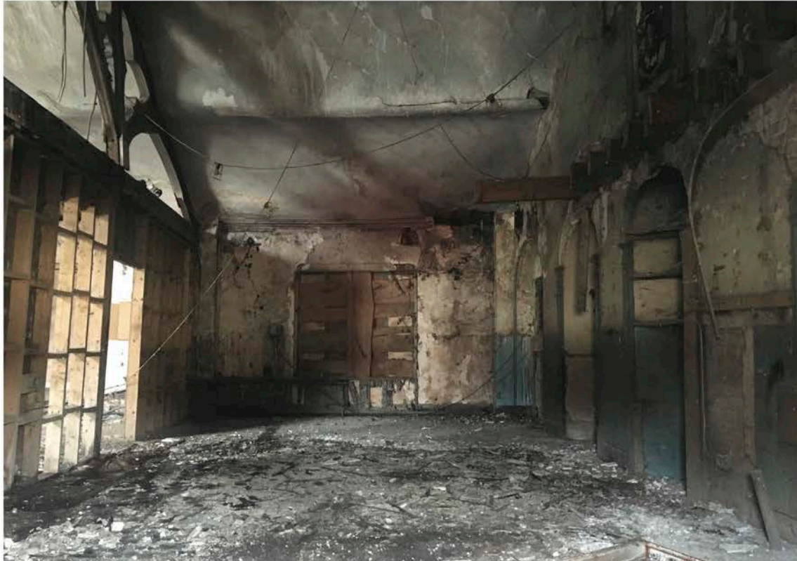
Current Condition of St. Patrick's Classical School.
