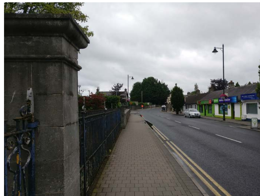
Photograph showing the wrought-iron railings and piers surrounding the forecourt of the former county offices Source : Architect's own.
