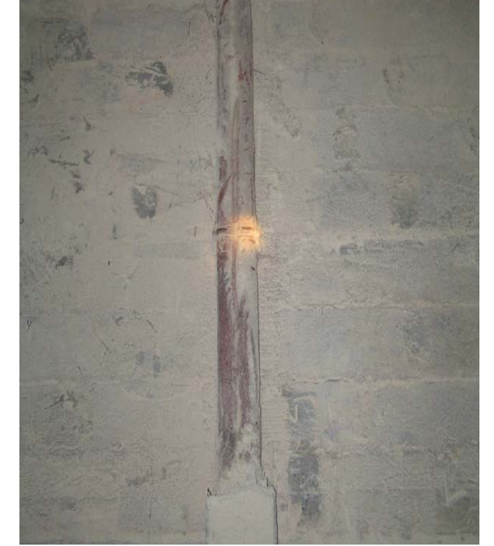
Original cast iron columns encased in concrete (Source: Con Kehely Study)
