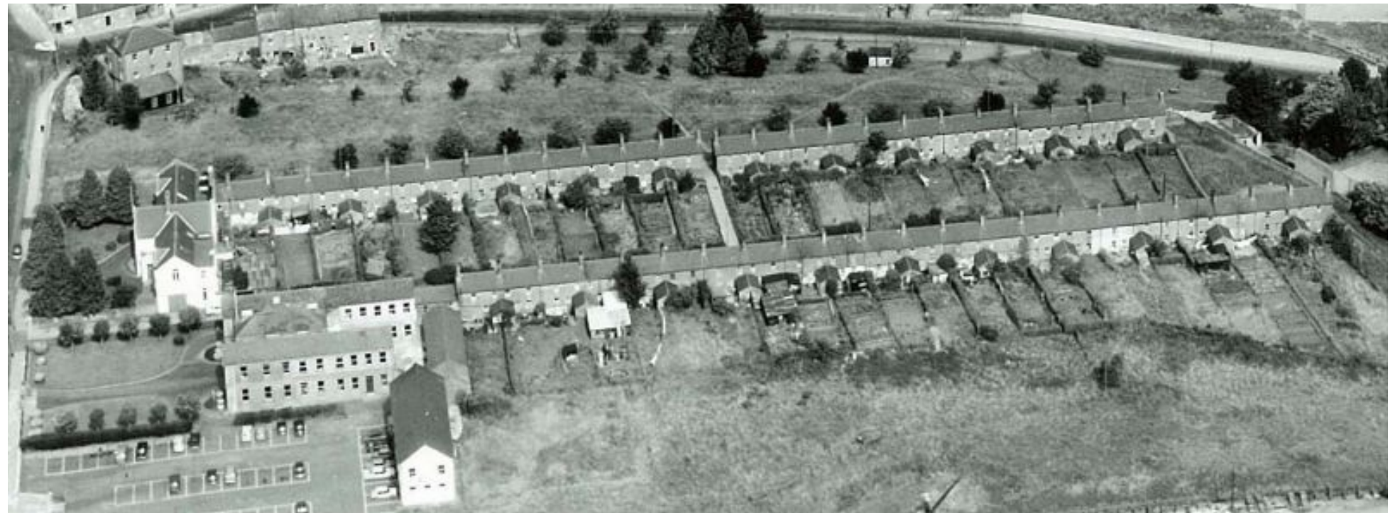
Historic Photography showing the County Council Offices, the two rows of St. Finian's terrace and the Irish National Foresters' Hall (site now occupied by Solstice Art Centre). Source: Navan Historical Society
