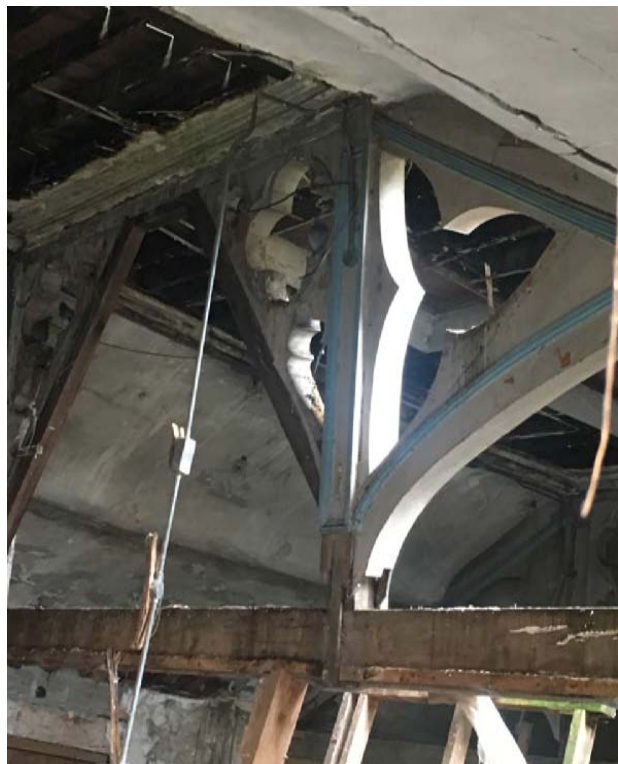
Decorated roof trusses.
