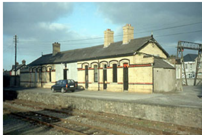
Detached nine-bay single storey Railway Station, 1885. Yellow brick facade with blue and redbrick strings at cill and impost levels.
