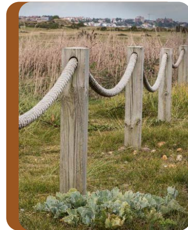
(E5) TIMBER POSTS AND ROPE FENCING
