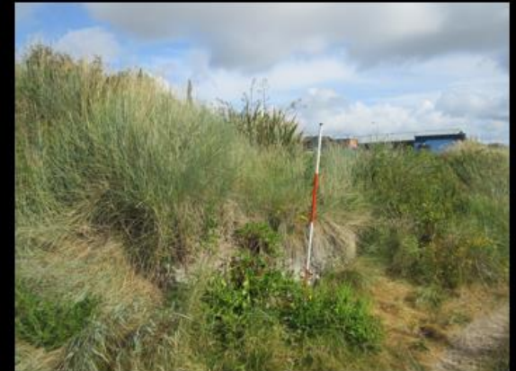
1930s Mass concrete wall buried in dune.
