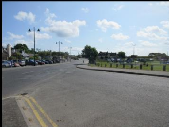
R150. Bus turning loop. Facing E
