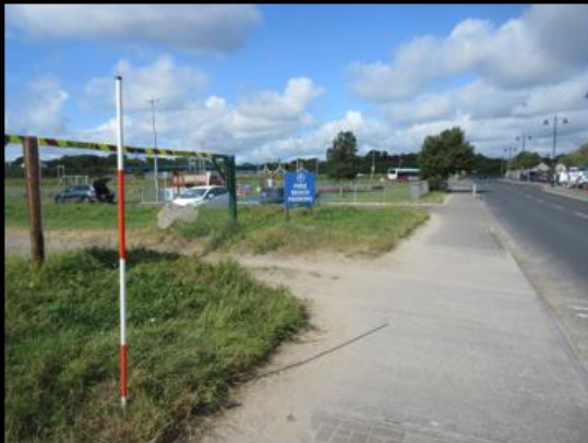
R150. Beach parking to Playground Parking. Facing W
