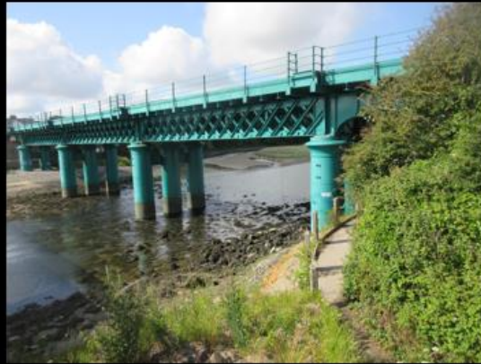
Railway viaduct. Facing SW
