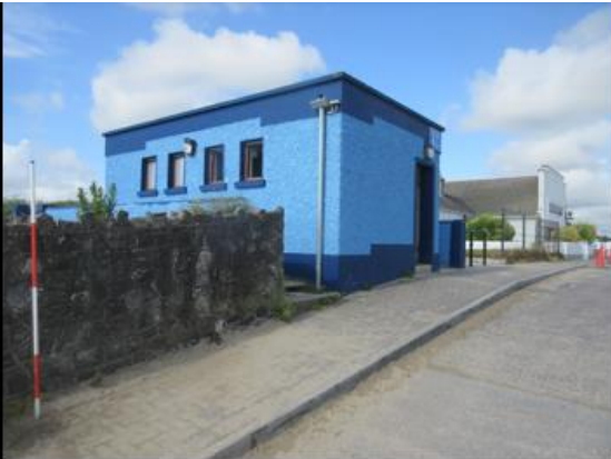
Public toilets on beach. Facing SW
