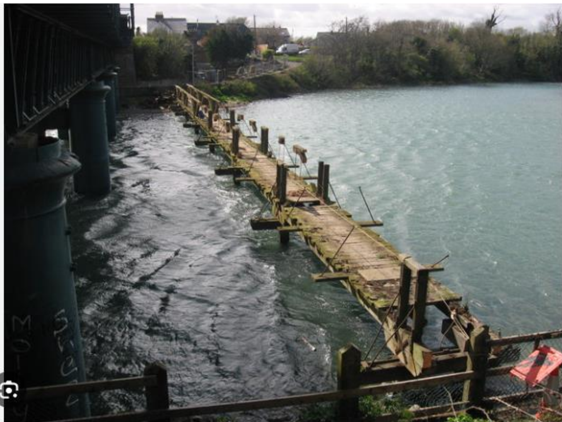
Demolition of Laytown footbridge © Kieran Campbell :: Geograph Ireland
